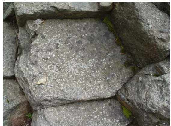
Rupnica, columns, view from above
