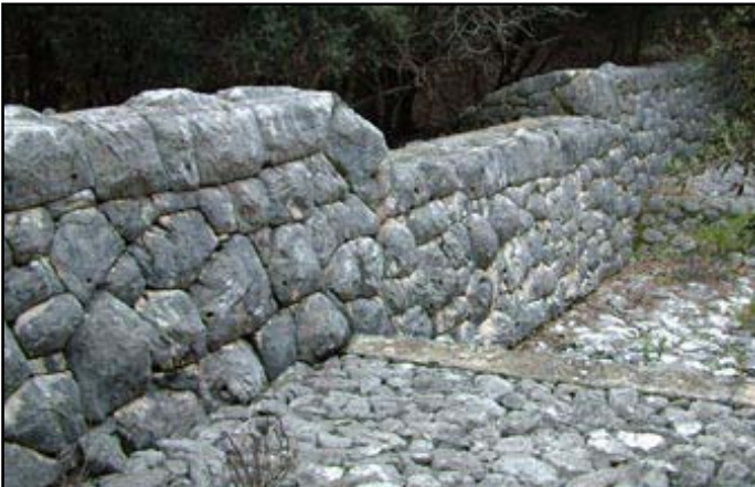
Fig. 34: Vela Draga retention dam.
