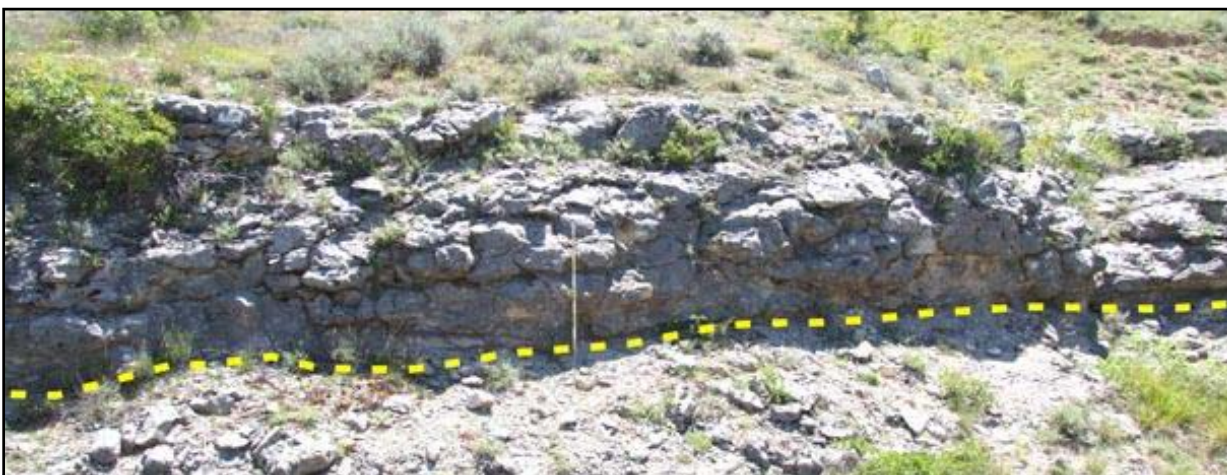
Fig. 71: The sandy siltstone bed and underlying at the bottom of the photo.
