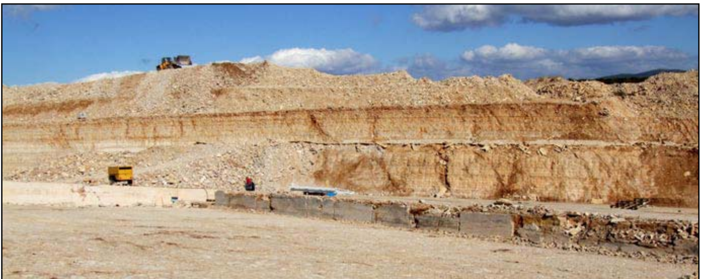
Fig. 29: Modern technology in “Kamen Benkovac” enables making the long vertical walls and opening the extensive bed surfaces.
