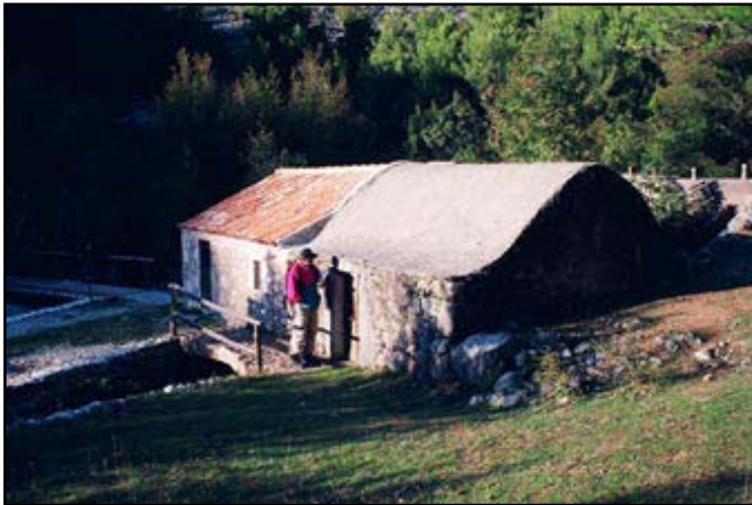
Fig. 21: Refurbished old water mill.
